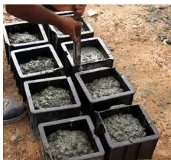
Fig. 6 Casting of Specimens
